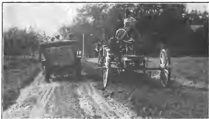
Working on New Road Which Leads to Winston-Salem
